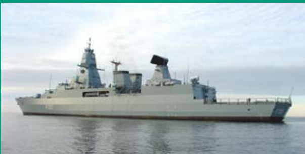
Maritime wastewater treatment for navy vessels
